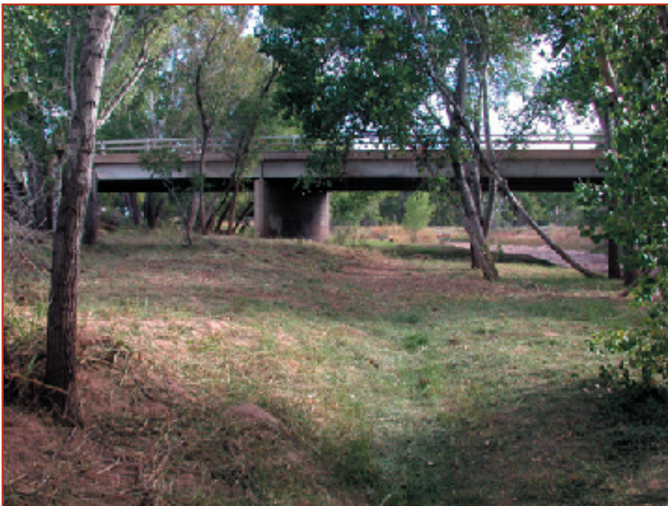
Looking at the finished product, an improved firebreak next to the bridge.
