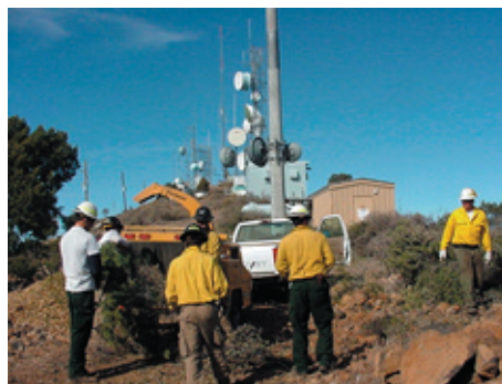
Firefighters chip brush, after using hand tools and chainsaws to clear around Guthrie Peak Communications Site.
