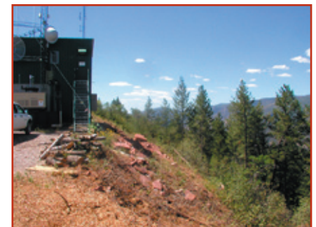
Communications site following treatment work.
