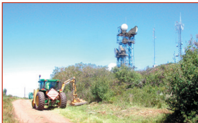
Garfield County mower clearing brush to create the fuel break.
