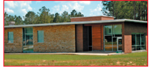
The new Southern Regional Fire Training Center in Pearl, Mississippi.
