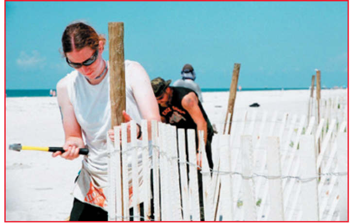
Hotshots working to build sand fence in southern Alabama.
