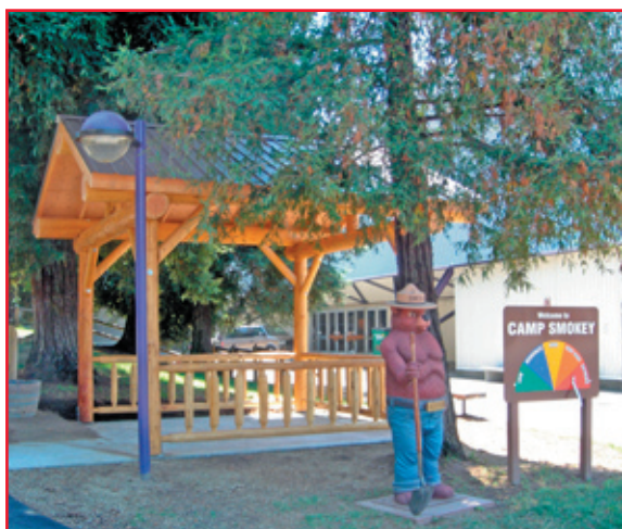
The Camp Smokey Command Post, built with small roundwood logs obtained from hazardous fuels projects in northern California.
