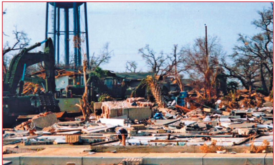
Crews arriving in Mississippi faced a monumental debris removal job as a result of Hurricane Katrina.
