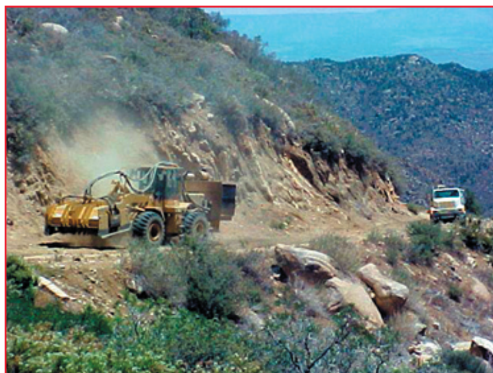
Road repairs on emergency access route in the Hualapai Mountains.
