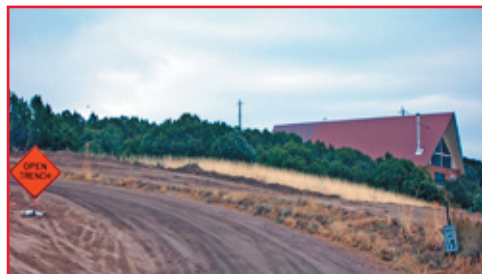
This home, in the wildland urban interface of Pocatello, is adjacent to new development that will fall under the new interface codes.
