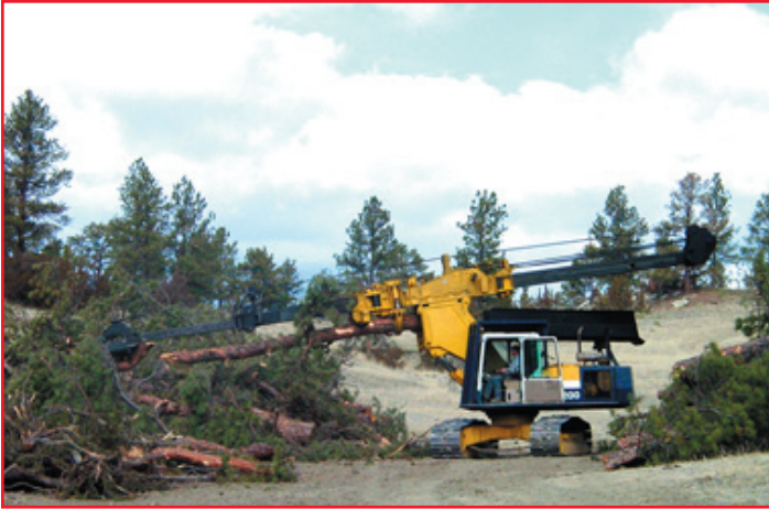
Mechanical equipment working on the Miles City area project.
