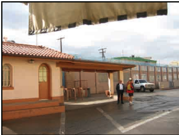
PHOTO 1 VIEW OF THE NOGALES EAST LPOE (SOUTHWEST VIEW)
