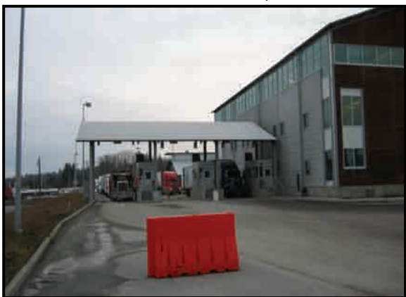
PHOTO 4 VIEW OF THE PACIFIC HIGHWAY LPOE (EAST VIEW)
