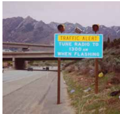
Figure 6.5. CommuterLink Highway Advisory Radio Sign
