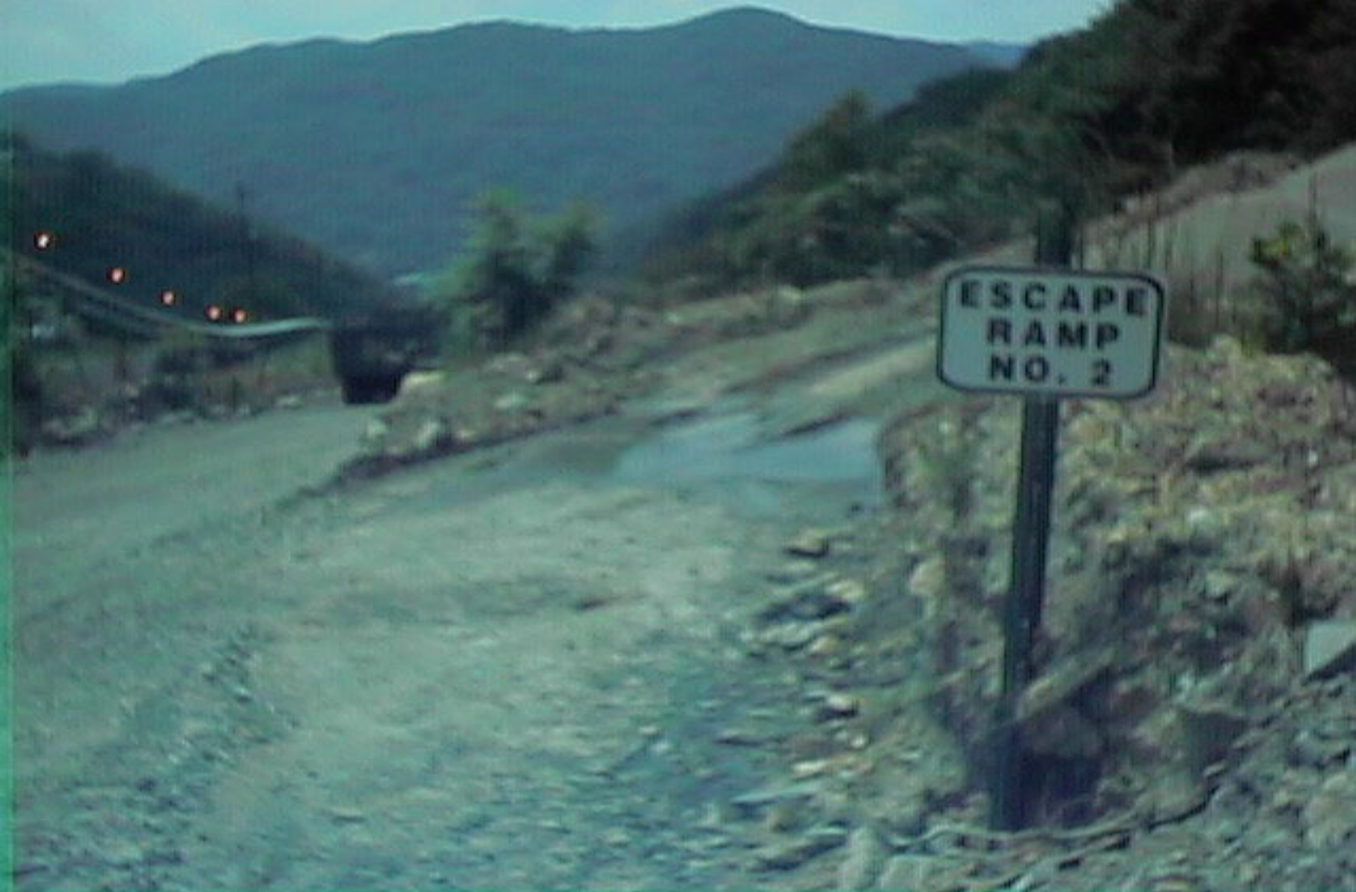
Three runaway-truck escape ramps had been constructed on the steep grade as a safety measure.
