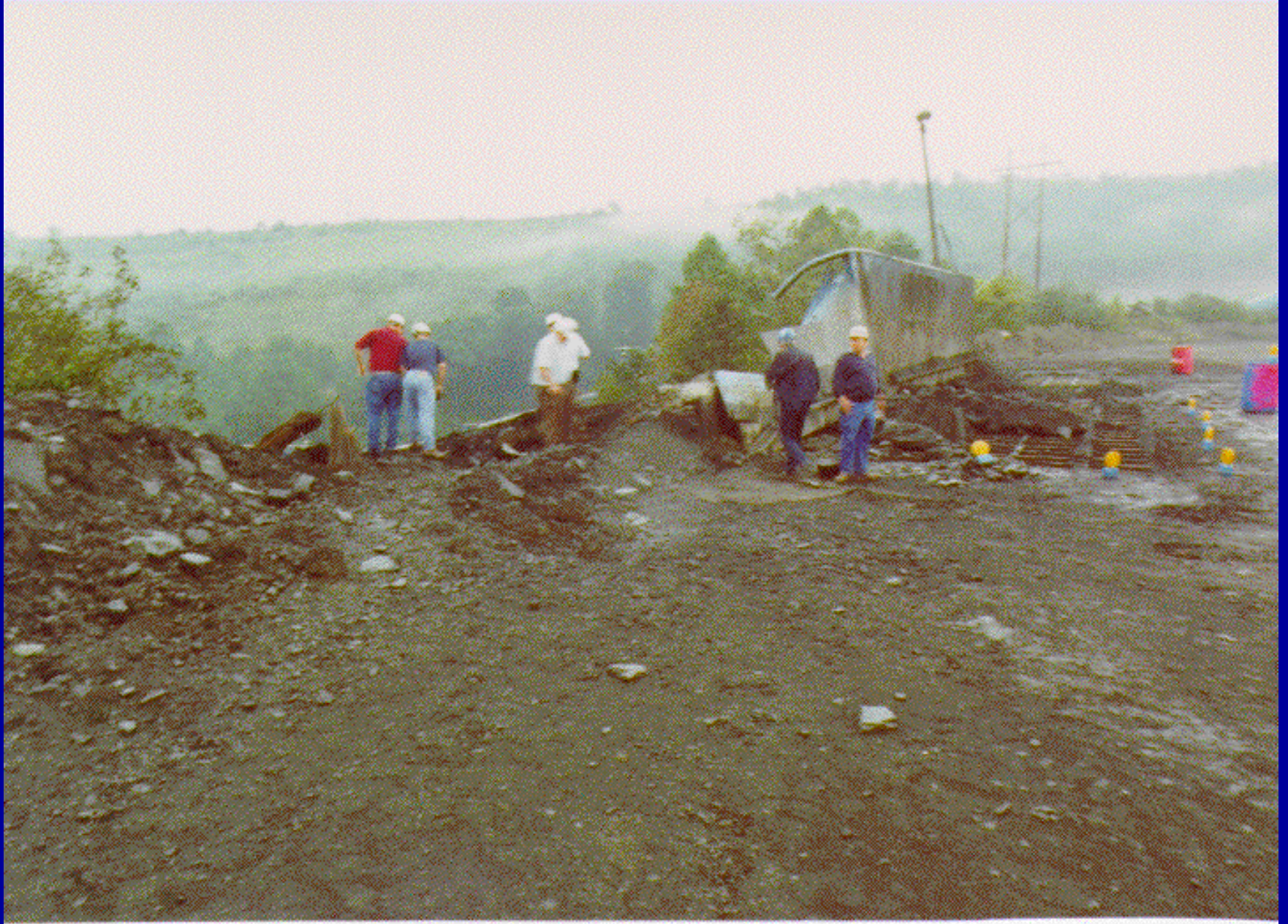
This is a close-up view of the area where the truck left the haul road...
