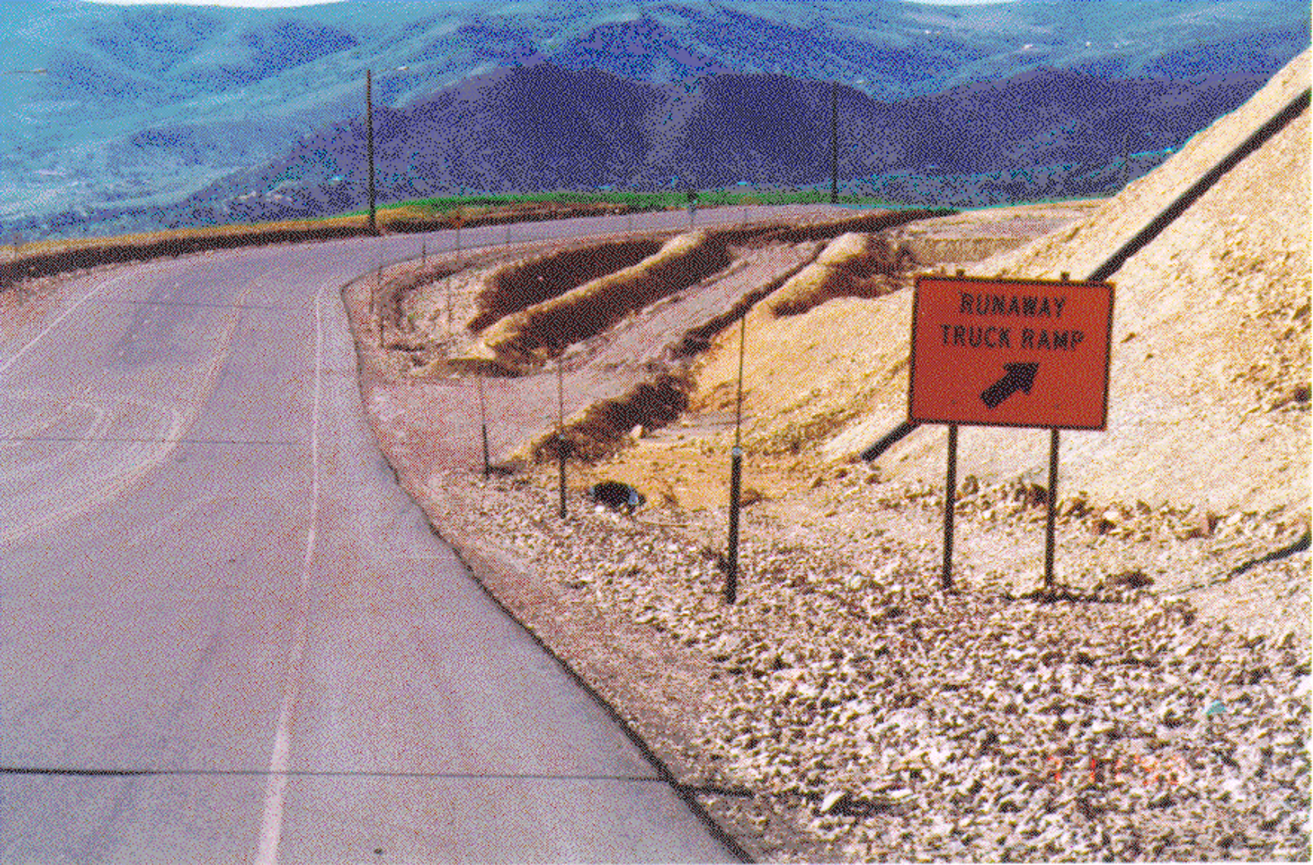
An example of a runaway escape ramp at a copper mine in Utah. A bed of loose gravel is used on the ramp to help bring a runaway truck to a controlled stop.
