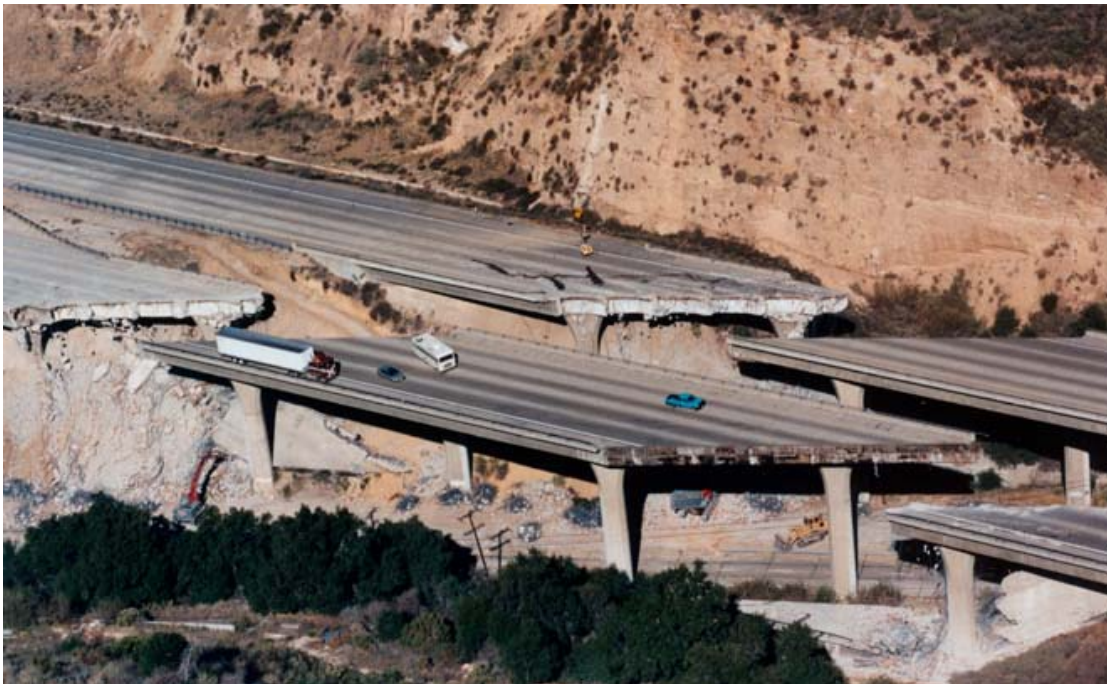
Figure 14. I-5 damage at Gavin Canyon (Source: Caltrans)
