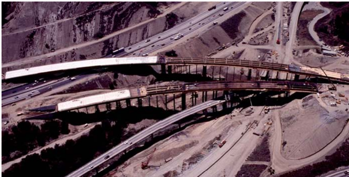
Figure 17. Reconstruction after the Northridge earthquake (Source: Caltrans)
