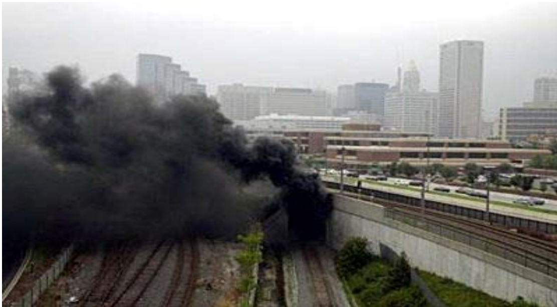
Figure 11. Smoke from the south portal of the Howard Street Tunnel (Source: Baltimore Sun )
