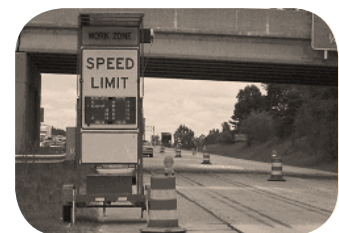
*Variable speed limit sign in a Michigan work zone. Photo courtesy of Michigan State University.
