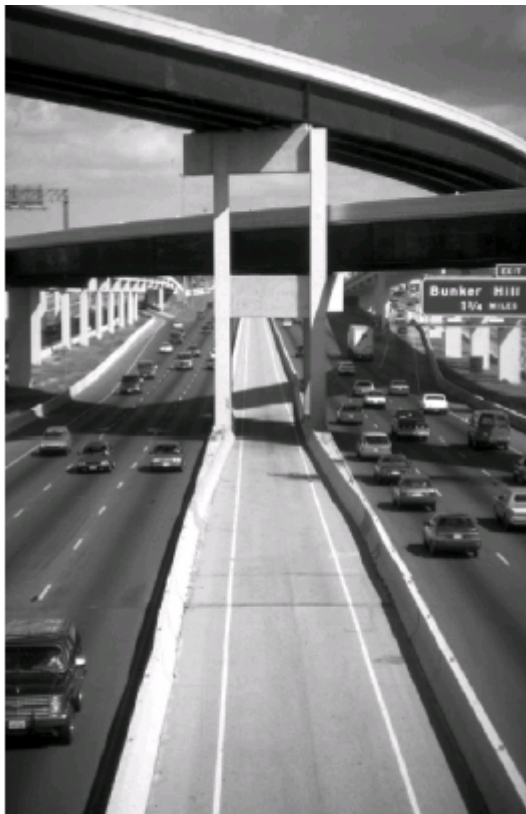
Figure 9-1: Examples of Exclusive / Barrier-separated HOV Facility (Reversible)
