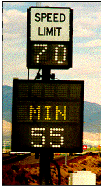
Figure 8-10: Variable Speed Limit Sign.
