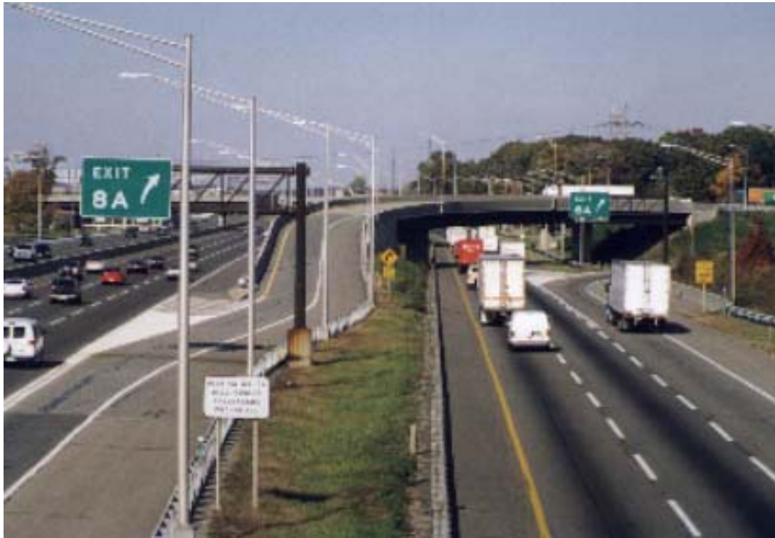
Figure 8-2: Dual-dual Section of New Jersey Turnpike.
