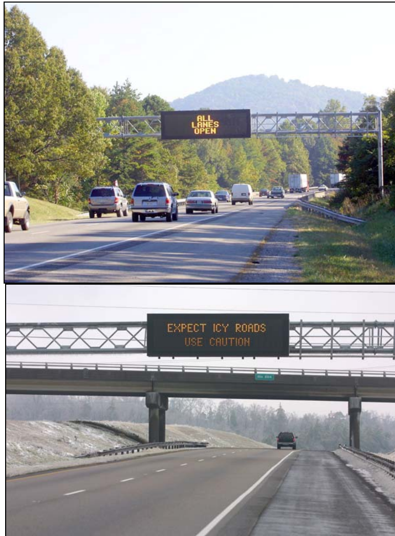
Figure 13-3: Examples of Light-Emitting Matrix CMS Technologies (Courtesy of Virginia DOT)
