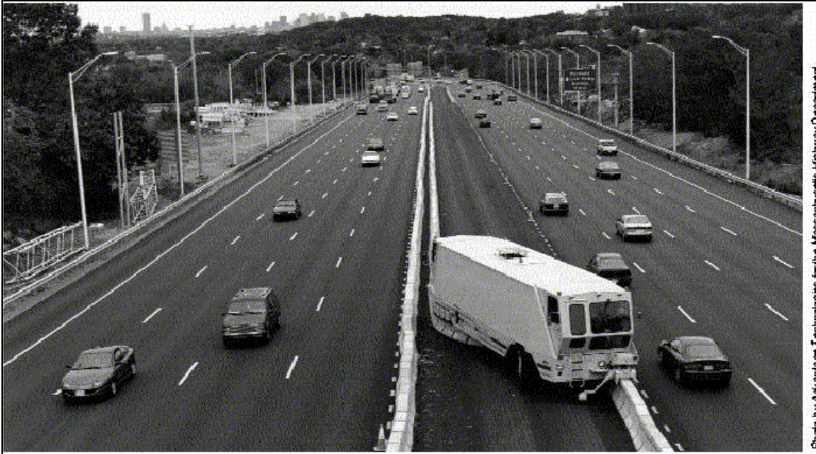
Figure 8-15: Moveable Barrier Being Repositioned
