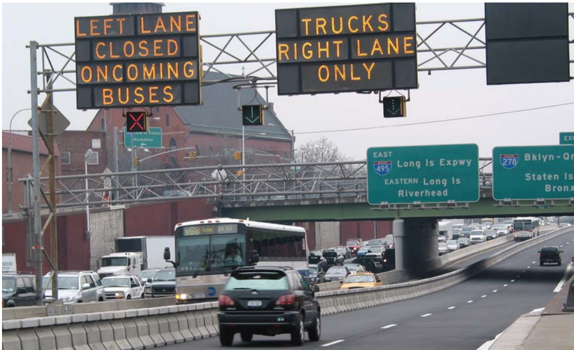
Figure 8-1: Example of Managed Lanes
