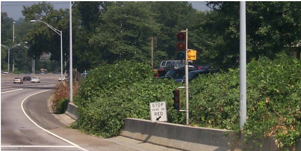
Figure 7-2: Ramp Metering Signals
