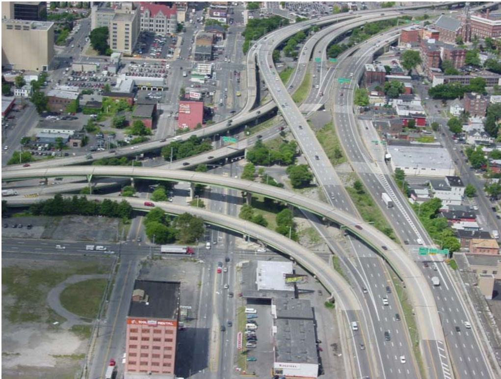
Figure 1-4: Freeway Interchange (I81 / I690 in Syracuse, NY)
