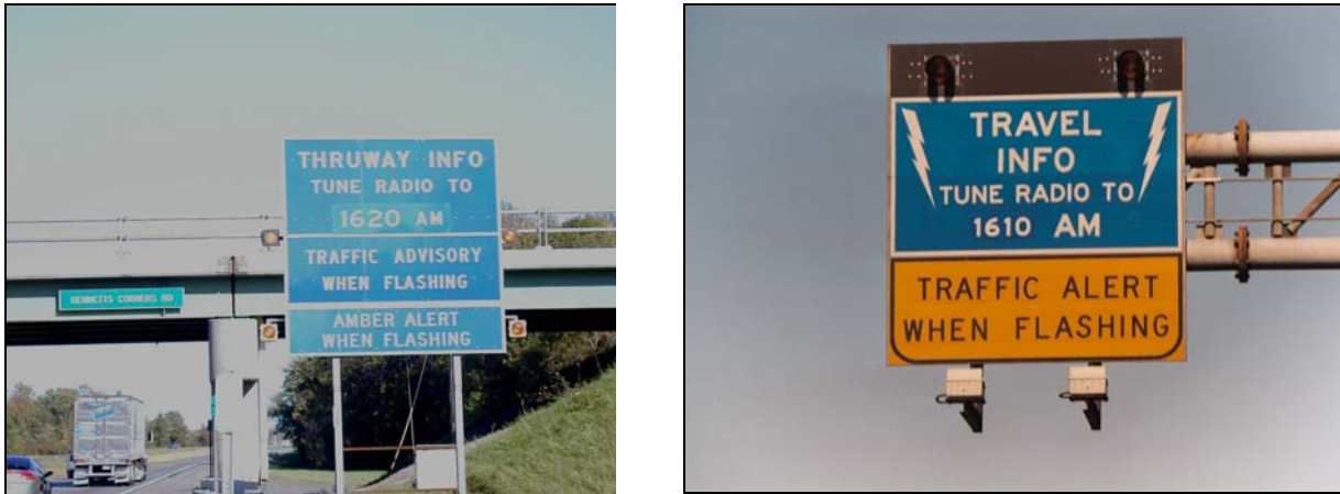
Figure 13-7: Highway Advisory Radio Sign
