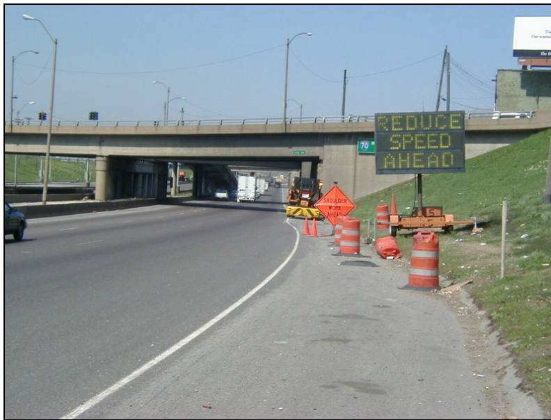
Figure 13-4: Portable CMS in Operation in a Work Zone
