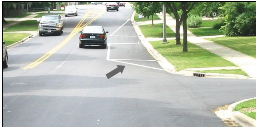
This photo depicts a “parking box” that prevents vehicles from parking too close to the intersection and obstructing the side street driver’s line of sight.
