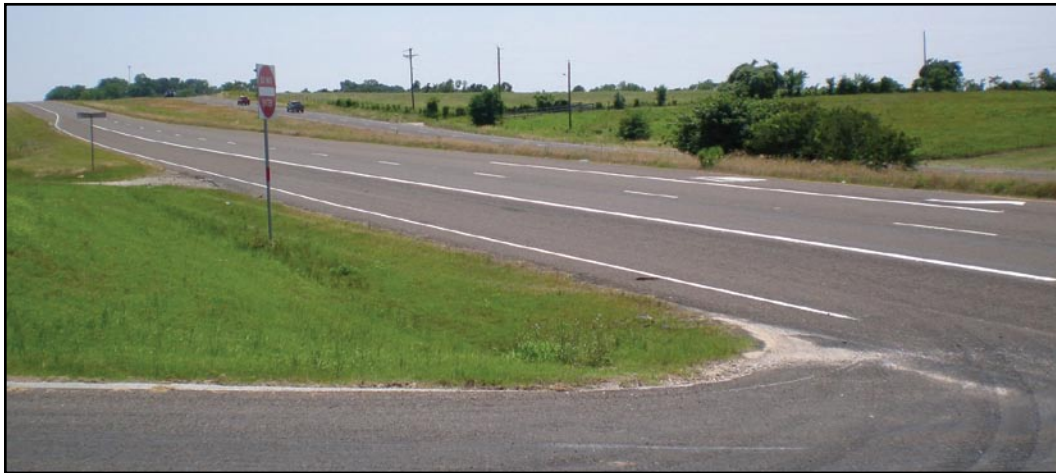
Photo by: Texas Transportation Institute
