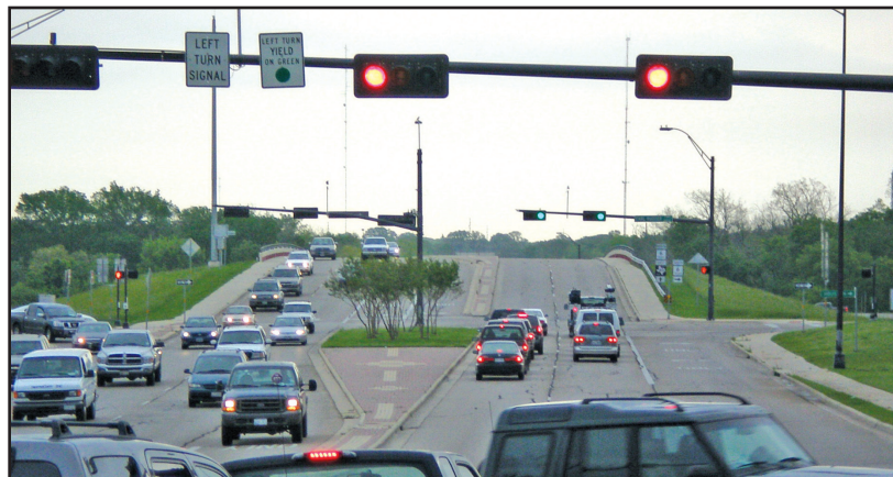
Photo by: Texas Transportation Institute
