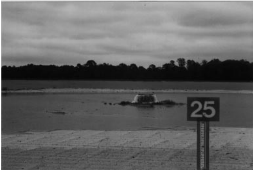
Figure 3. Reclaimed water application to rapid infiltration basin.
