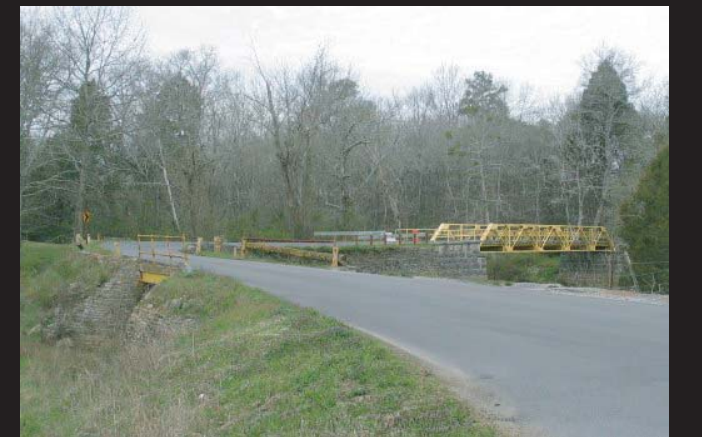
Slough & Alexander's Bridges
