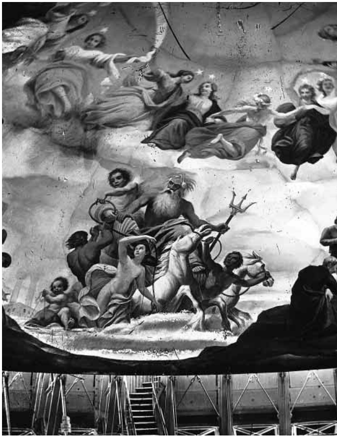
Fig. 9–14. Early photograph from the balcony. This photograph of “Marine” shows how the space under the canopy perimeter was left open, so that light could be reflected onto the fresco from the windows in the dome. The balcony was enclosed when the Rotunda was air conditioned in the 1940s. Brady-Handy Collection, Library of Congress.
