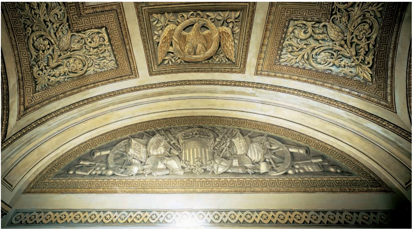
Fig. 6–33. Area with trophy lunettes and ceiling with illusionistic coffers. The original tempera decoration of the ceiling remains mostly untouched. Near S–111 and S–139.
