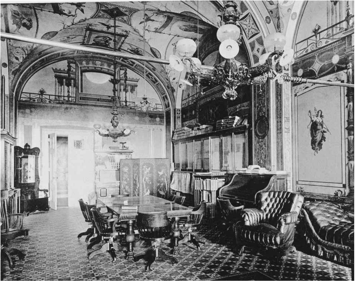
Fig. 6–13. Room S–127 as it appeared c. 1900. By the turn of the century, Brumidi’s murals were partially obscured by bookcases and other furniture. Note the original bronze chandeliers decorated with anchors.
