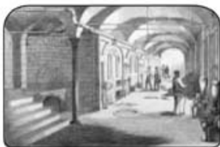
"Basement of the Houses of Congress, showing the extensive heating apparatus for warming the buildings," June 1858 U.S. Senate Collection
