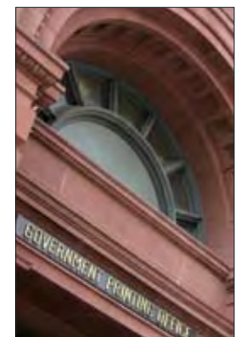
GPO entrance on North Capitol Street, NW.
