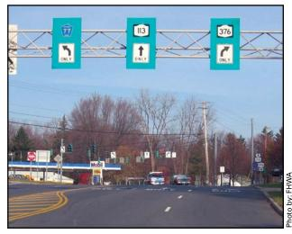
While this photo shows lane assignment signing at a signalized intersection, a similar strategy can be used at complex unsignalized intersections.
