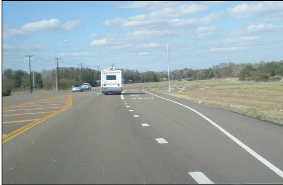
Photo by: Texas Transportation Institute
