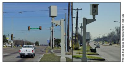
These photos show the front and rear of a typical red light camera installation.
