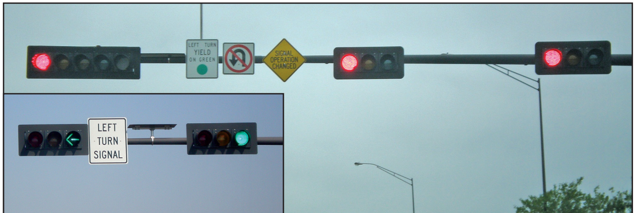
Photos by: Texas Transportation Institute, FHWA
