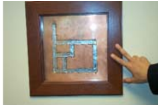
Betrusted Data Center construction, using copper-lined walls with soldered edges to reduce RF Emissions
