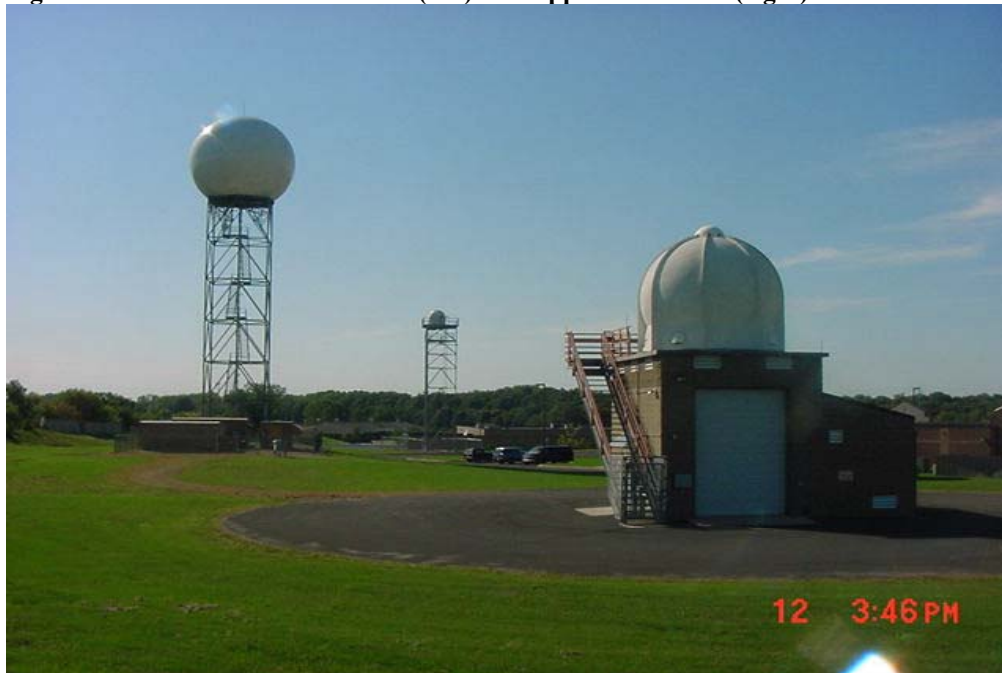
Figure 3: Chanhasen WFO Radar (left) and Upper Air Tower (right)
