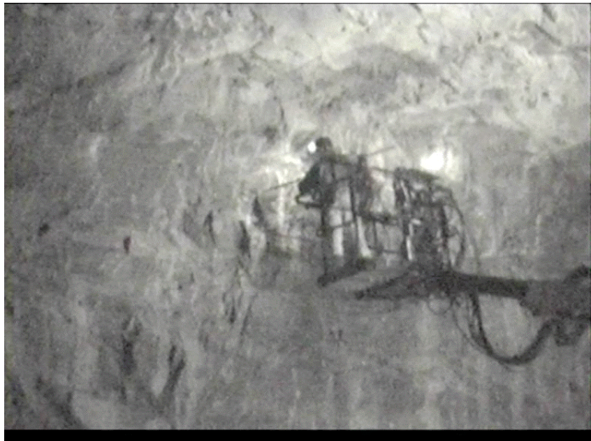
Photograph 15 – Illumination of the Back and Roof with Two Halogen Lights Installed on the Cab Roof of a Lift
