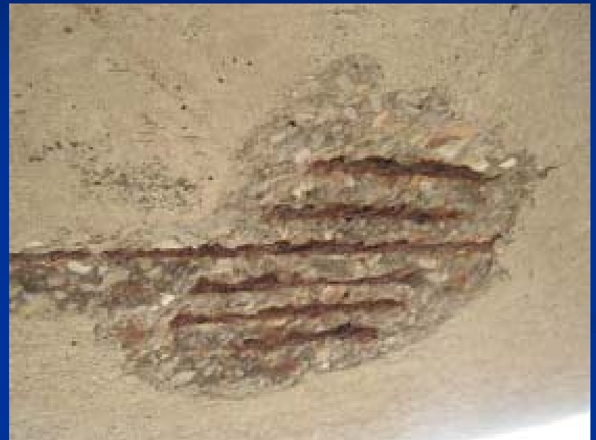
Corrosion Damage
