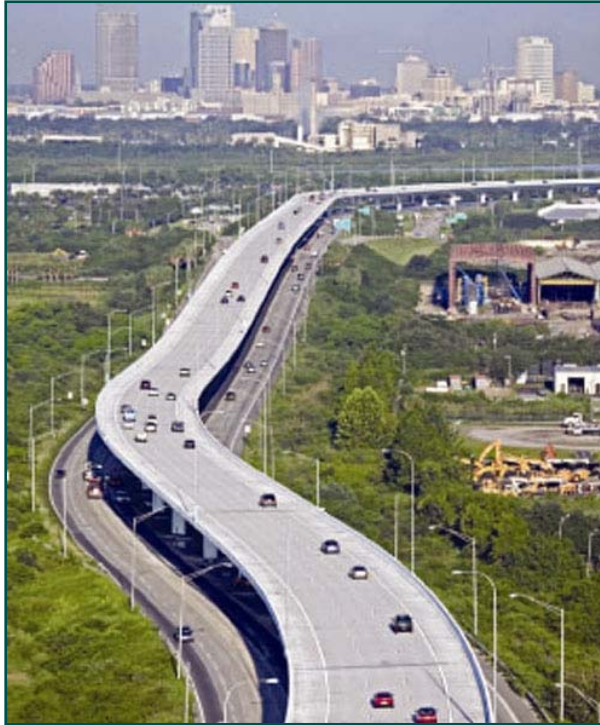
Lee Roy Selmon Expressway Reversible Lane Viaduct Tampa, Florida
