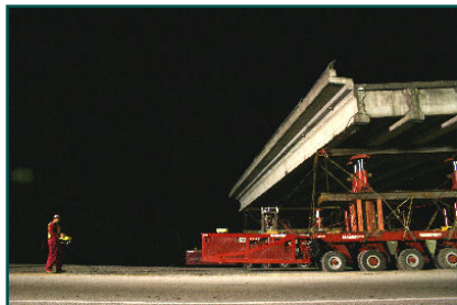
Keep America Moving During Bridge Construction
