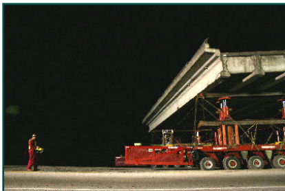
Keep America Moving During Bridge Construction
