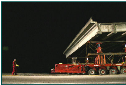
Keep America Moving During Bridge Construction
