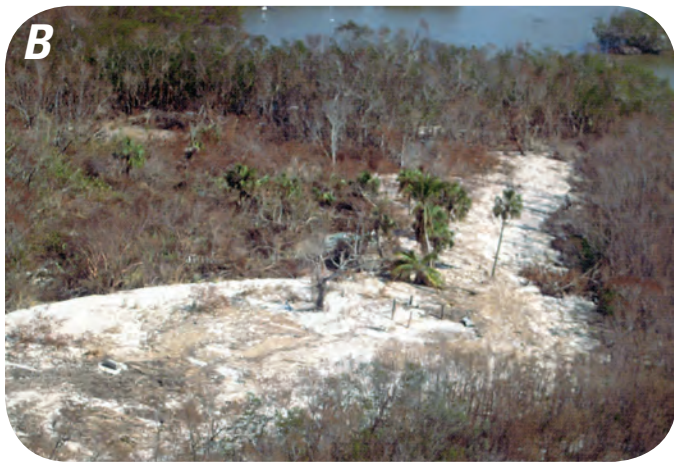
Figure 4. Lostmans River Ranger Station (LRS) in Florida in January 1998 (A), well after Hurricane Andrew (which hit in 1992), and in October 2005 (B), just after Hurricane Wilma.
