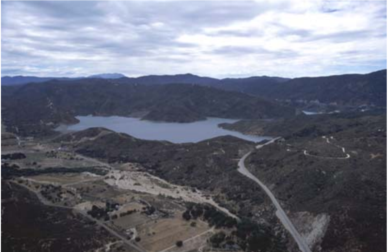
Figure 13. Summit Valley. Aerial view of Summit Valley and the Silverwood Lake region. Cedar Springs Dam is visible to the left. Horsethief and Little Horsethief Canyons drain into Summit Valley, which is visible below the lake and dam. Historically, arroyo toads were documented in the vicinity of Cedar Springs and the region that is underneath the lake.
