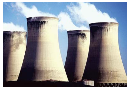
Nuclear Power Plant Cooling Towers
