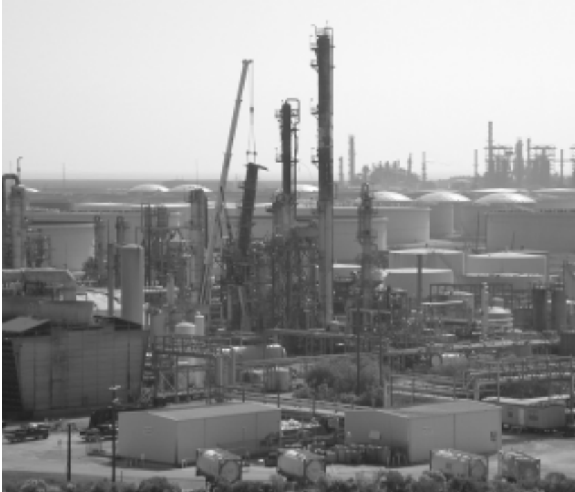
Figure 1. Facility overview. (Note: The crane is attached to the column damaged in the explosion.)
