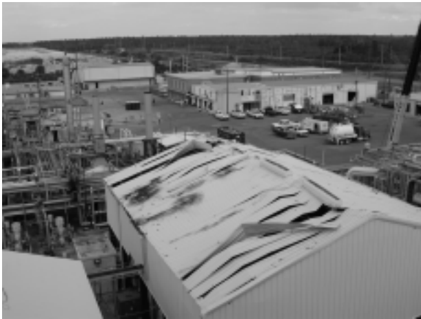
Figure 9. Damage to control room roof and door.
