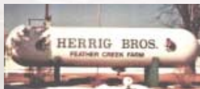
Herrig Tank before Explosion
