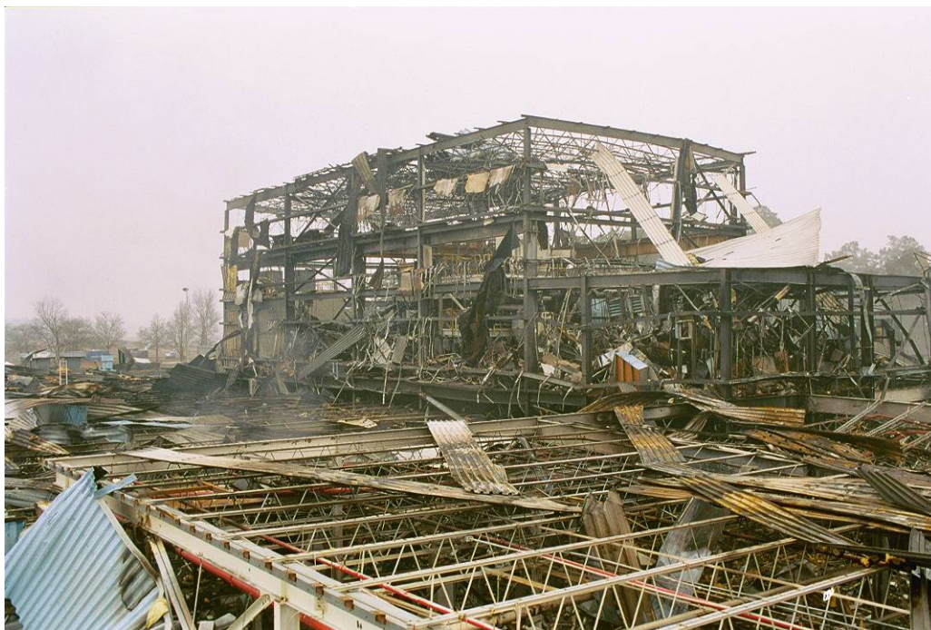
Figure 4. West Pharmaceutical Services facility destroyed by polyethylene dust explosion 13
