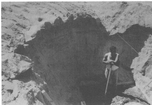
Figure 7—Installing the concrete foundation for one of the Ismailia lysimeters.
