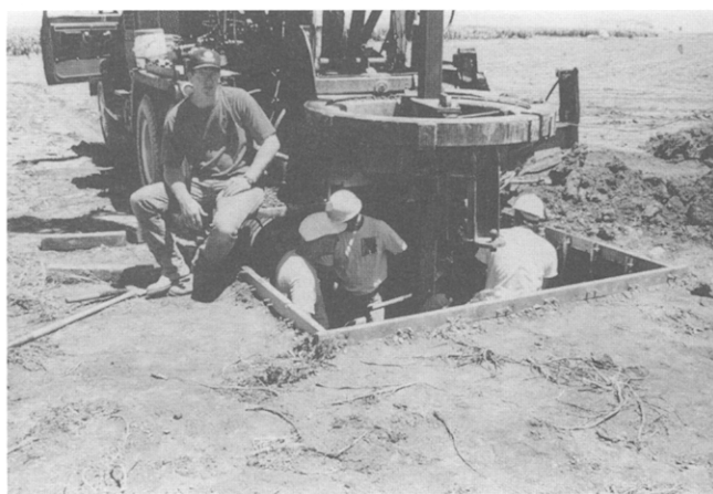
Figure 5—Excavating for the foundation and enclosure for the Bushland lysimeter.
