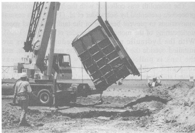
Figure 4—Lifting the Bushland soil monolith from the ground for overturning.
