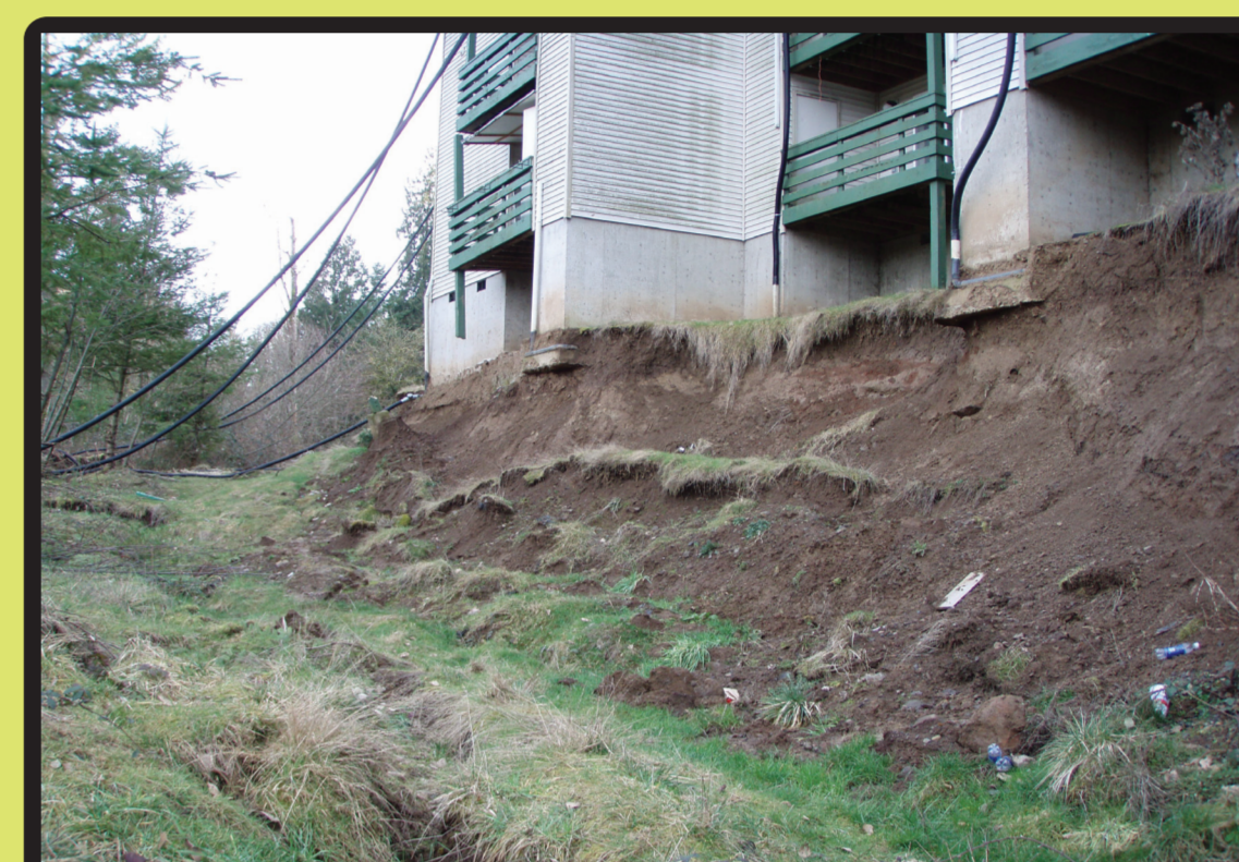
Photograph depicting scarps along the crest of the toe of the large Newell Creek Apartments landslide - 2007.
