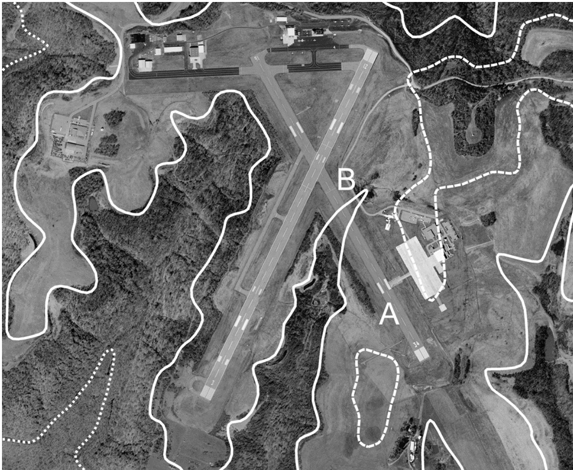
Figure 2. The outcrops of the Pittsburgh, Waynesburg, and Washington coals, derived from the 1966 vintage topography of the Tiltonsville 7.5-minute quadrangle (U.S. Geological Survey, 1997b), are superimposed on a 2003 image of the Wheeling-Ohio County Airport. The dashed line represents the original outcrop position of the Washington coal. The Washington was initially surface mined at location A in the mid 1940s to make room for the runway alignment. The Waynesburg has also been surface mined adjacent to the runways during the 1980s. The dotted line represents the outcrop of the Pittsburgh coal. Subsequently all three coals were extensively surface mined, and the land has been returned to the original contour so the outcrop lines approximate those of the 1940s. The 1:62,500 Wheeling 15-minute topographic map (U.S. Geological Survey, 1902) was also useful in deciphering the excavation and mining history of the area.
