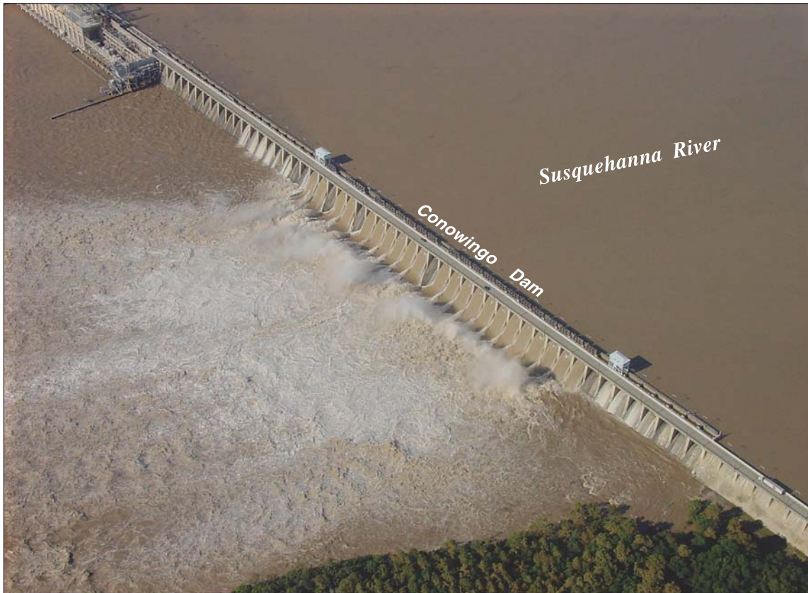
Photograph showing the release of water from the Conowingo Dam on the Susquehanna River in Maryland, September 21, 2004 at 10:00 AM as a result of Hurricane Ivan. When this photograph was taken, discharge at the Susquehanna River near Conowingo, Maryland (USGS station number 01578310) was 348,000 cubic feet per second. (Photograph courtesy of Wendy McPherson, USGS).
