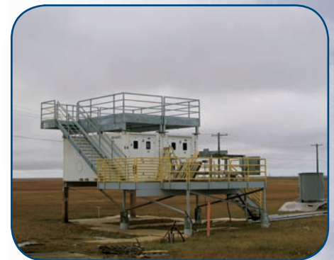
In September, installation was completed on the new Guest Instrument Facility in Barrow to provide additional instrument space and ease crowded working conditions.
