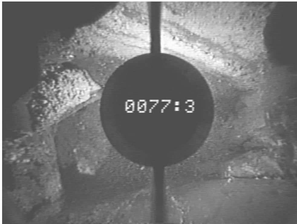
Figure 12. Images from borehole television survey showing fractures in well CC-2, Malvern TCE Site, Chester County, Pennsylvania. (A) 65.2 feet below land surface. (B) 77.3 feet below land surface. (C) 100.4 feet below land surface.
