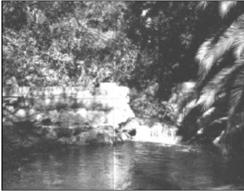
Figure 15. Photograph of Stenner Creek, Fish Barrier ST-2-1B.
