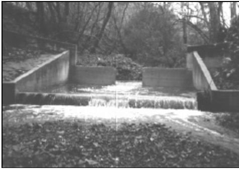
Figure 17. Photograph of Stenner Creek, Fish Barrier ST-2-3B.
