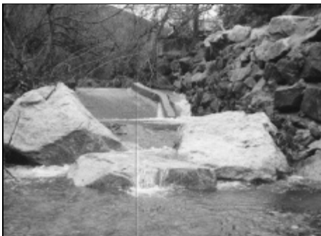
Figure 18. Photograph of Stenner Creek, Fish Barrier ST-3-1B
