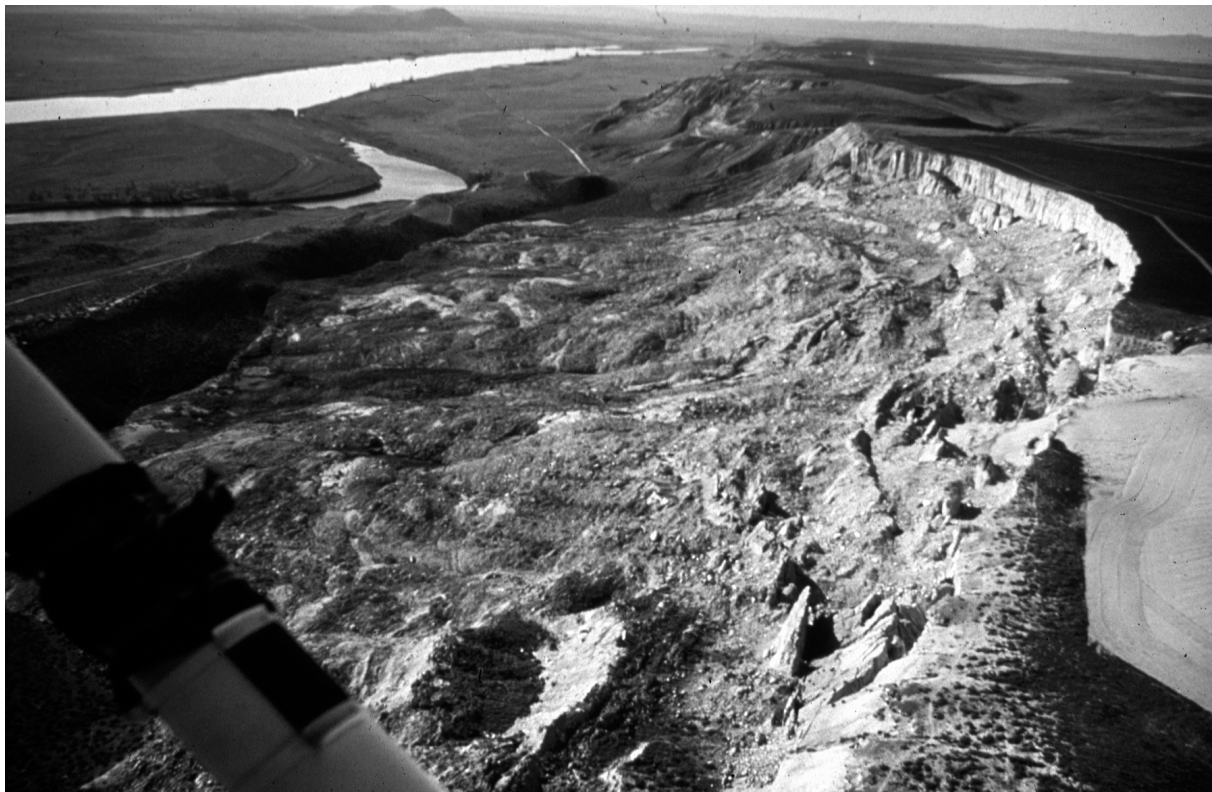
Fig. 25. April 1981 aerial oblique view of the 12-million-m 3 , irrigation-induced Savage Island landslide on the Columbia River, south-central Washington State, U.S.A. In the spring of 1981, hundreds of baby cliff swallows were killed when their nests in the 25-m-high main scarp were destroyed because of catastrophic headward recession of the landslide to the location shown.
