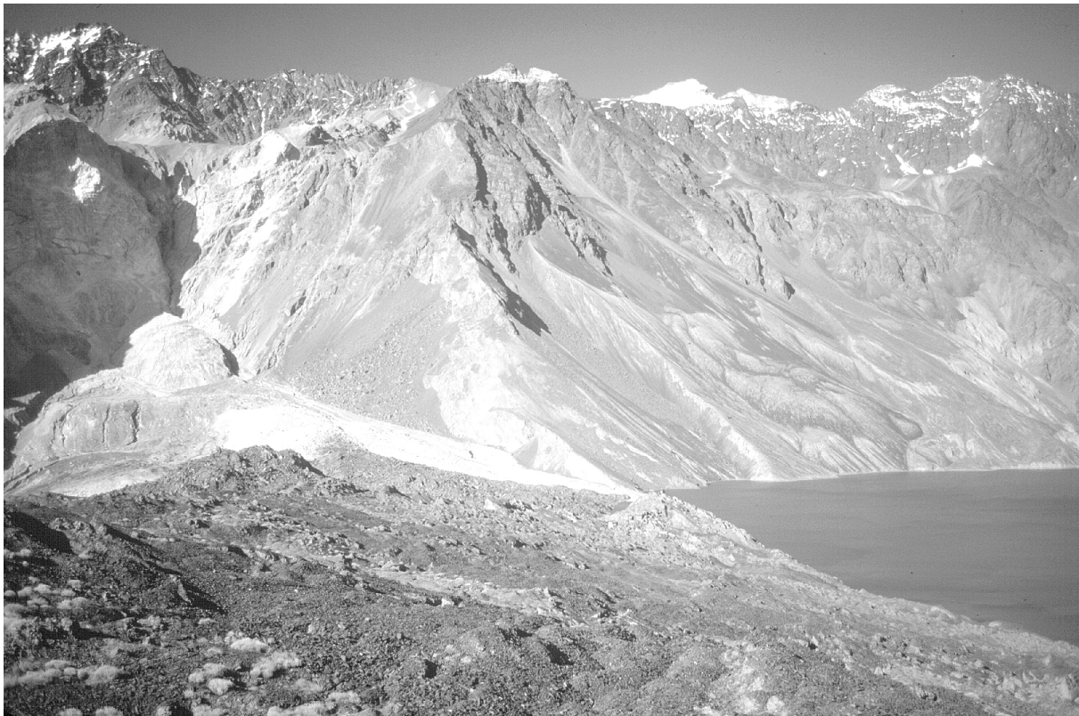
Fig. 12. View of Usoi landslide dam (foreground) and downstream (west) end of Lake Sarez., southeastern Tajikistan. Source area of the landslide is in the distance at the far left. (Photo by S. F. Cunha, Humboldt State University, Humboldt, California.)
