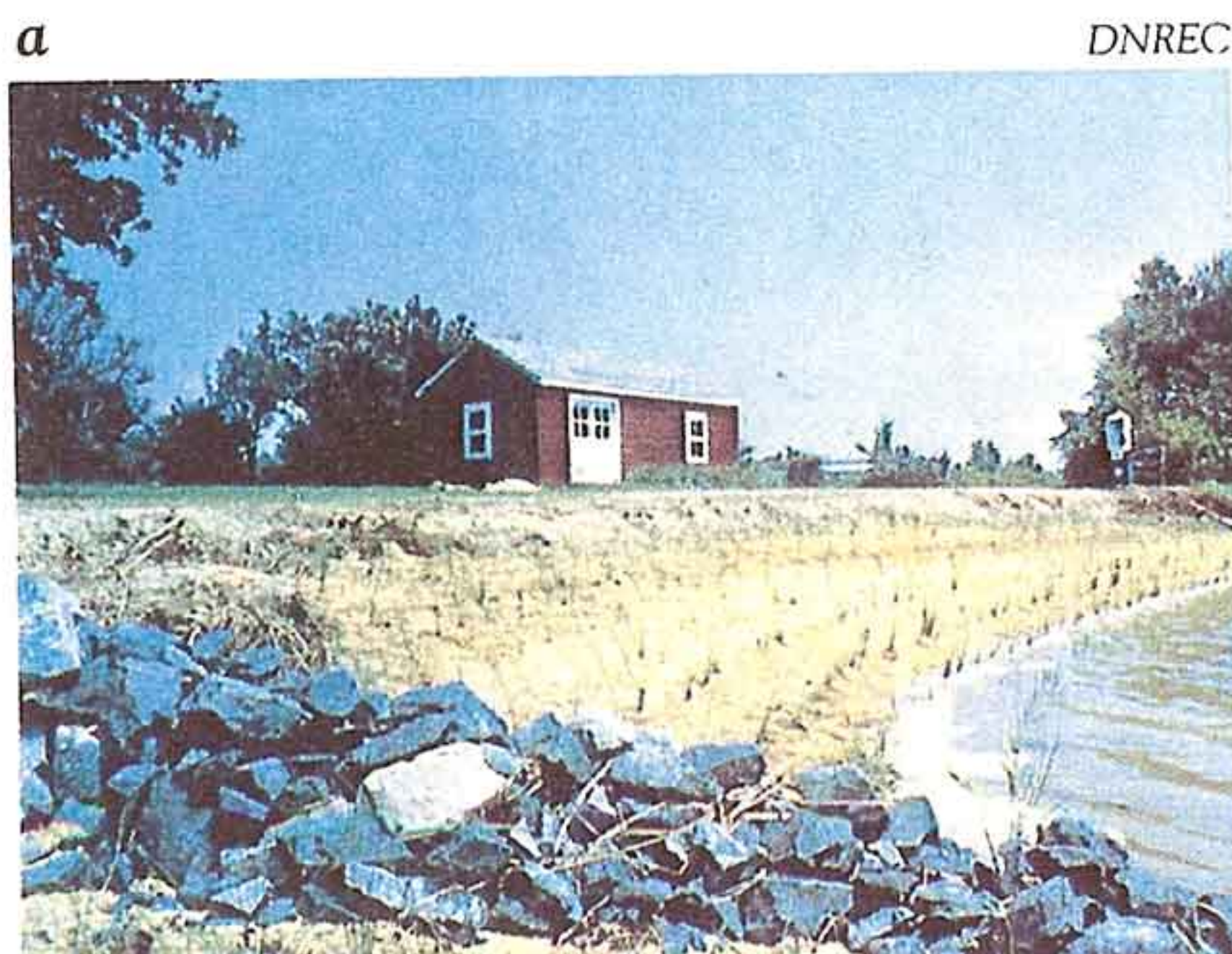
A fringe of marsh grasses as narrow as eight feet can reduce wave energy by over 50 percent (a—during planting; b—one year later).
