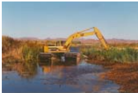
Digging out common reed to rehabilitate Imperial Refuge wetlands
